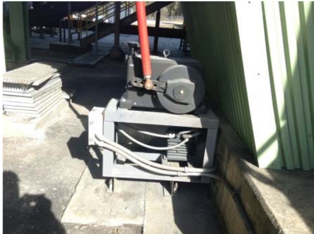
Figure A. Image of the FD damper actuator during 2015 audit. Note the position ~50%.
