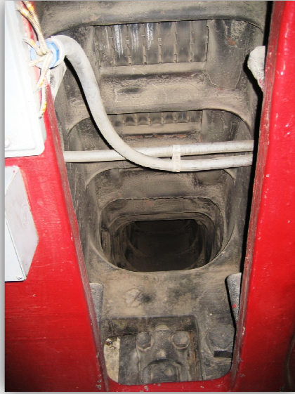
Figure 3 Long Lake dam generator passage for cooling air.
