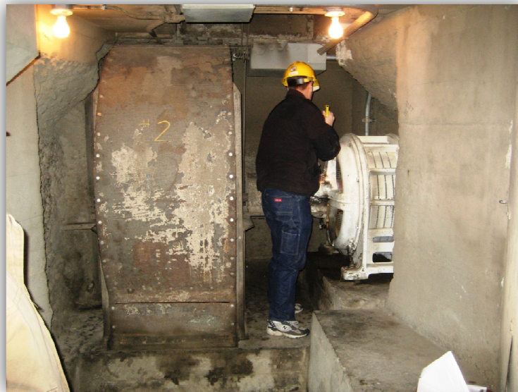
Figure 4 Long Lake stator cooling blower (left) and motor (right).
