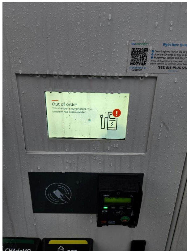
Figure 22: DCFC station with out of order error displayed on user interface (U/I) screen
