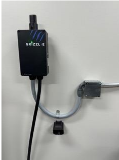
Figure 6: Residential charger installation
