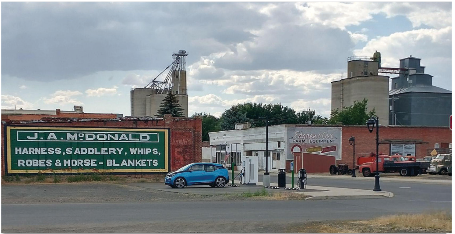
ABB Terra 184 DCFC in Sprague, WA
