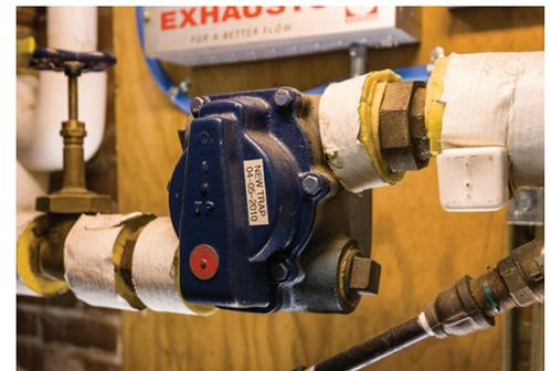
A rebuilt steam trap.
