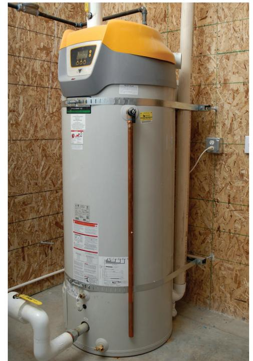
New 98% efficient natural gas water heater.
