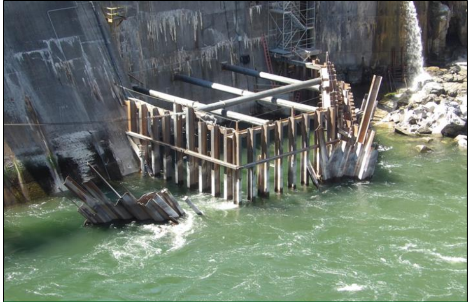
Damage to the temporary cofferdam during spring runoff along two walls where both the exterior and interior sheet pile cells were separated from the structural framework.
