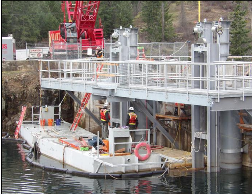
Fishway siphon platform installation on the forebay of Cabinet Gorge Dam.
