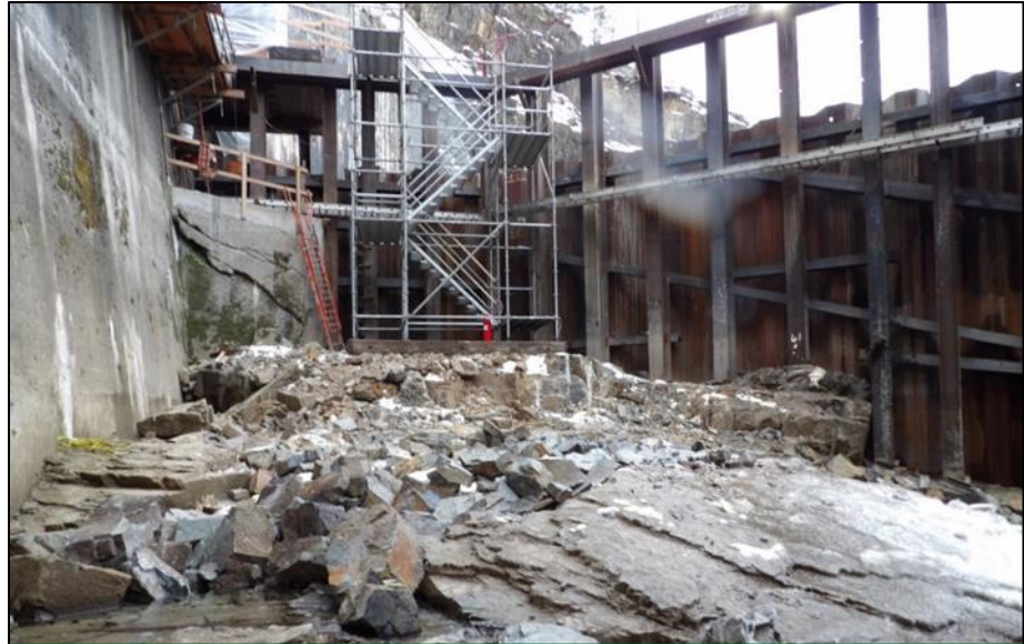
View from inside the cofferdam looking at bedrock to be removed for construction of the Fishway structure prior to spill.
