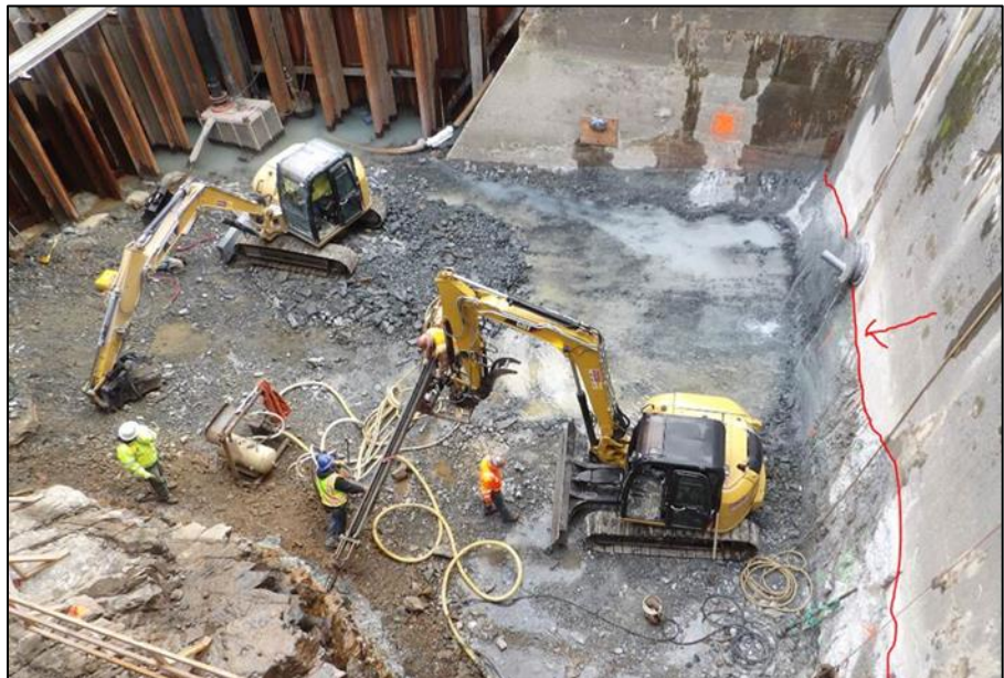
Excavation and rock dowel installation. Note, the red line denotes the concrete-bedrock interface.
