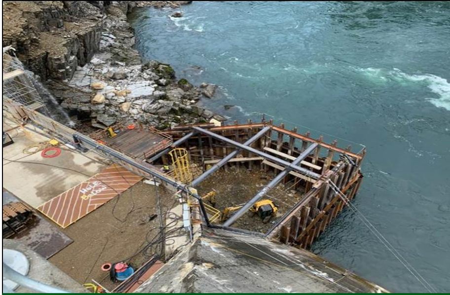
Overhead view of repaired cofferdam and rock excavation work.
