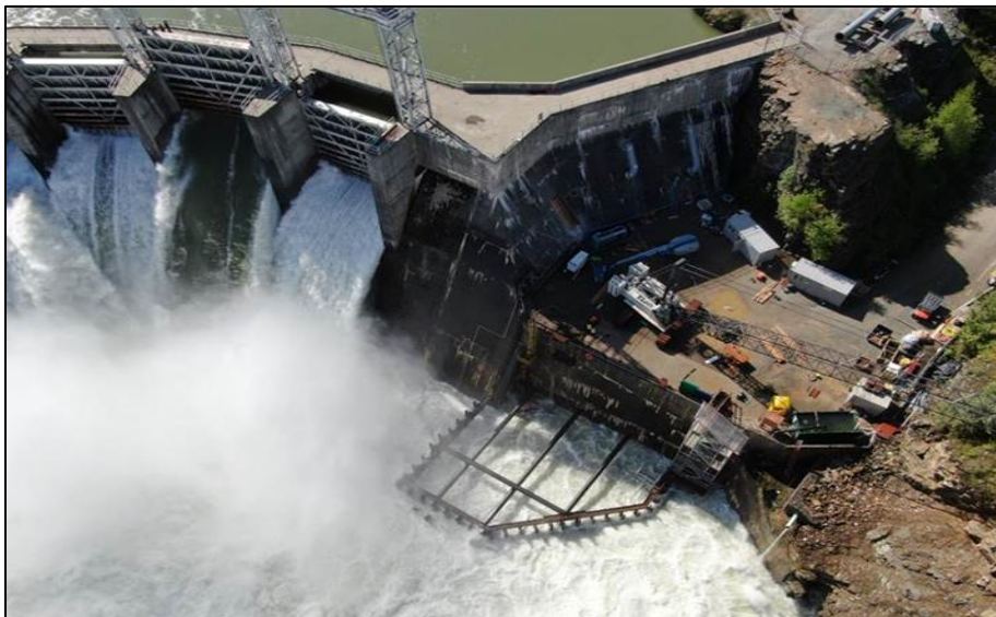
Cofferdam during spill at Cabinet Gorge Dam.
