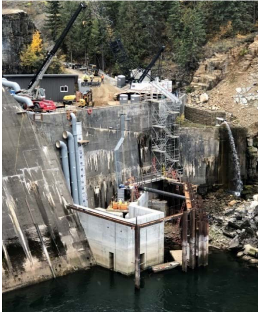
Removal of the cofferdam surrounding the CGDF construction site.
