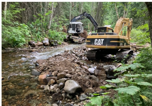
The Trestle Creek work focused on moving the creek channel away from the road and creating slow water habitat for juvenile Bull Trout.
