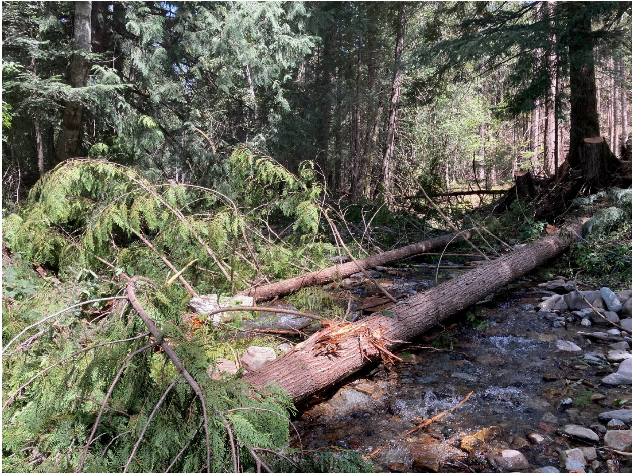
FIGURE 6. Trees felled for instream wood structure as part of phase I of the Trestle Creek Improvement Project.
