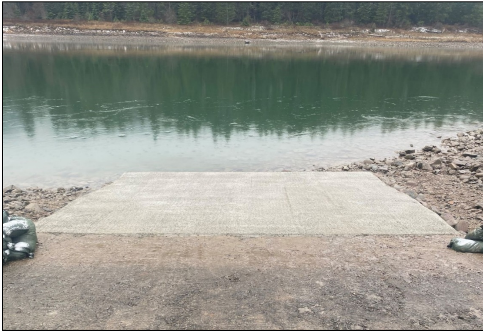
FIGURE 1. Sixteen-foot concrete ramp extension at the Thompson Falls State Park November 2021.
