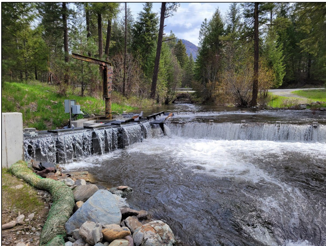
Figure 2. Graves Creek permanent weir trap overtopping as a result of clogged panels and trap box.
