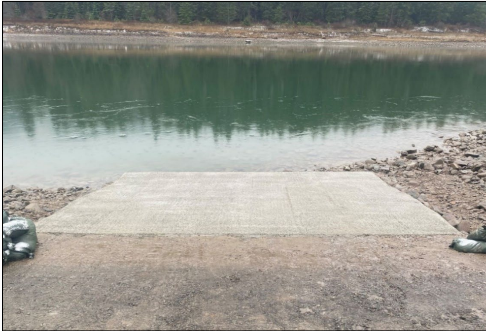
Figure 1. Sixteen-foot concrete ramp extension at the Thompson Falls State Park November 2021.
