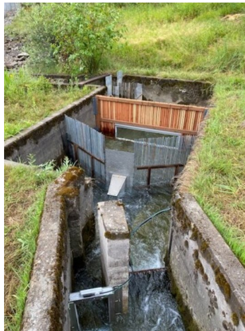
Cabinet Gorge Hatchery Ladder Trap including experimental elements for evaluating FRD performance.
