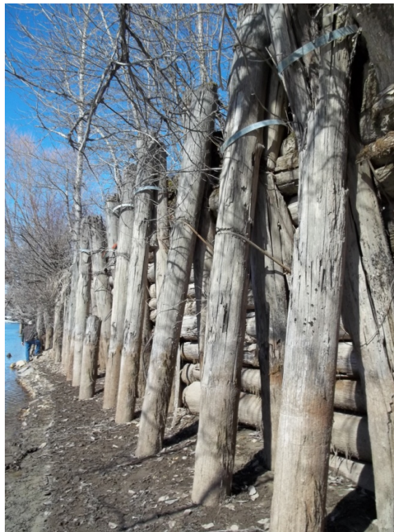
Photographs of the timber crib at the Shadowy St. Joe Log Landing Site.
