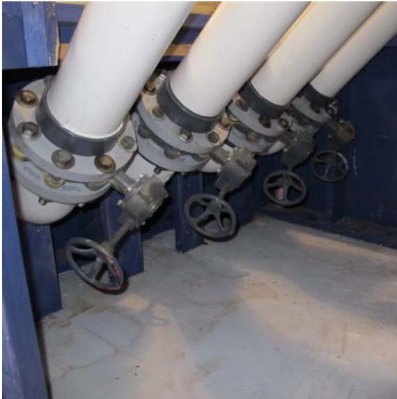
**Photo 5:** Values used to control the individual discharge for each powerhouse unit.
