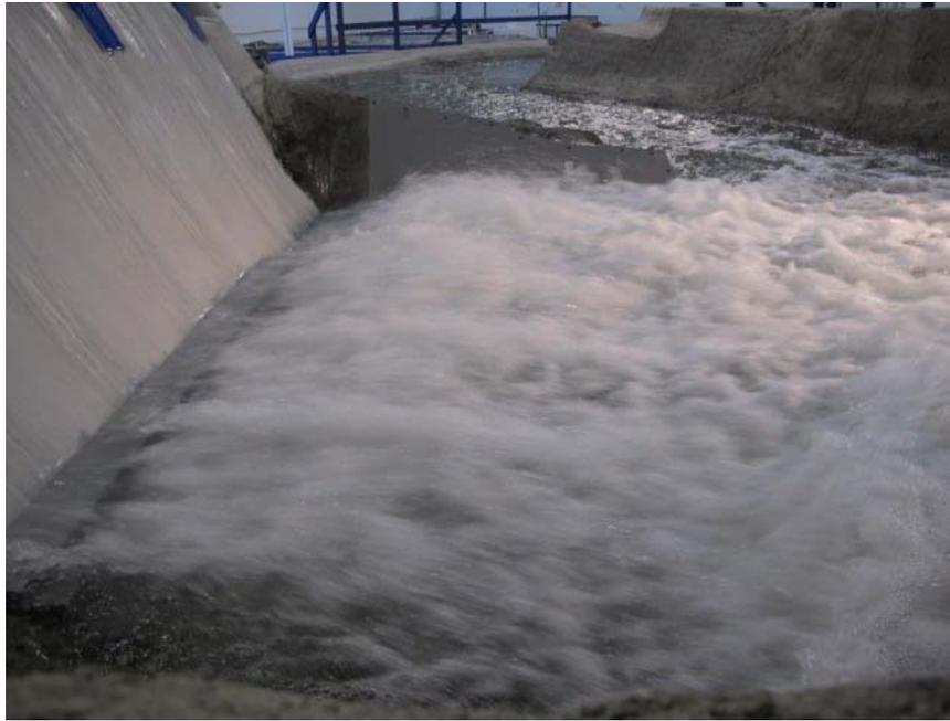
**Photo 7:** 20,000 cfs Spillway Discharge – Bays 3-8 – skimming (Bays 3-6), ramped surface jet (Bays 7 & 8)
