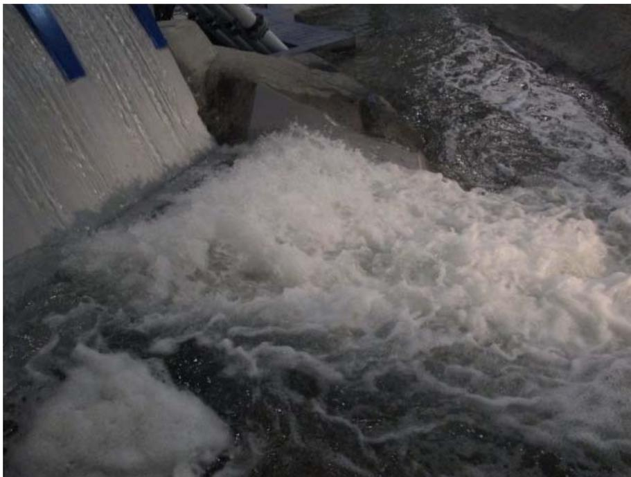
**Photo 2:** 25,000 cfs Spillway Discharge – Bays 5-8 – ramped surface jet flow regime.
