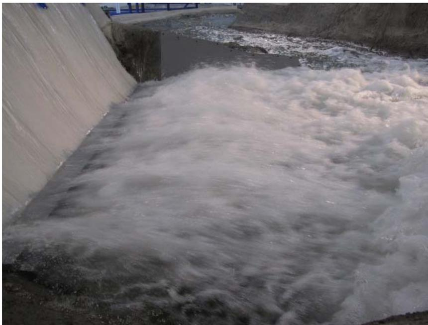
**Photo 8:** 25,000 cfs Spillway Discharge – Bays 3-8 – ramped surface jet (degrees varies).
