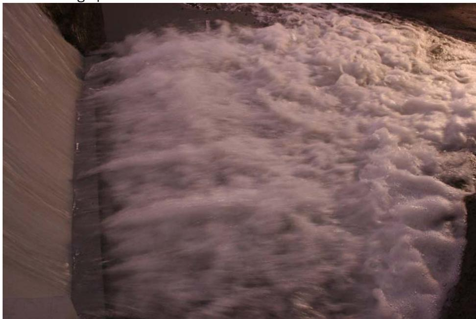
**Photo 2:** 25,000 cfs Spillway Discharge – Bays 3-8 – skimming and ramped surface jet flow
