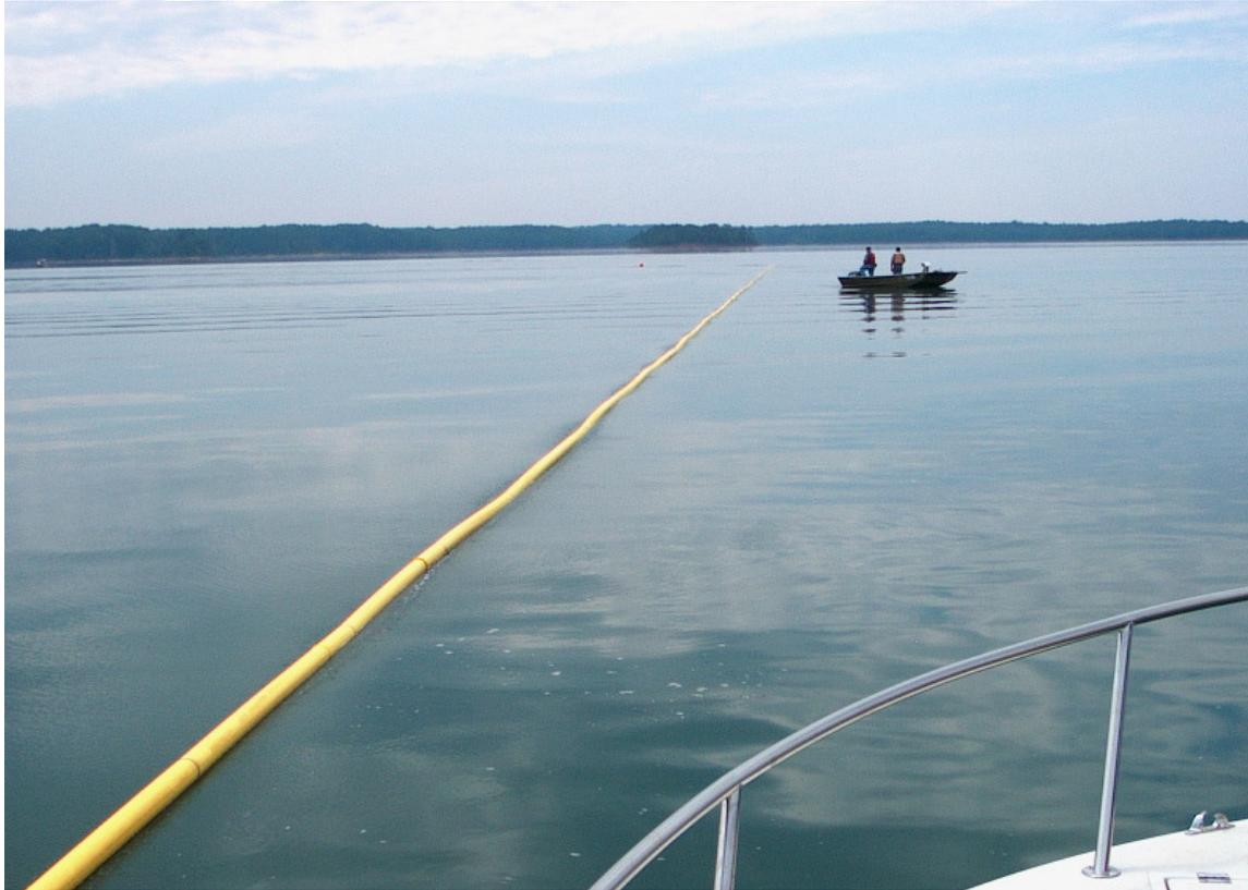
**Figure 5-2. Installation of Diffusers at Richard B Russell (US Army Corps of Engineers, 2002)**
