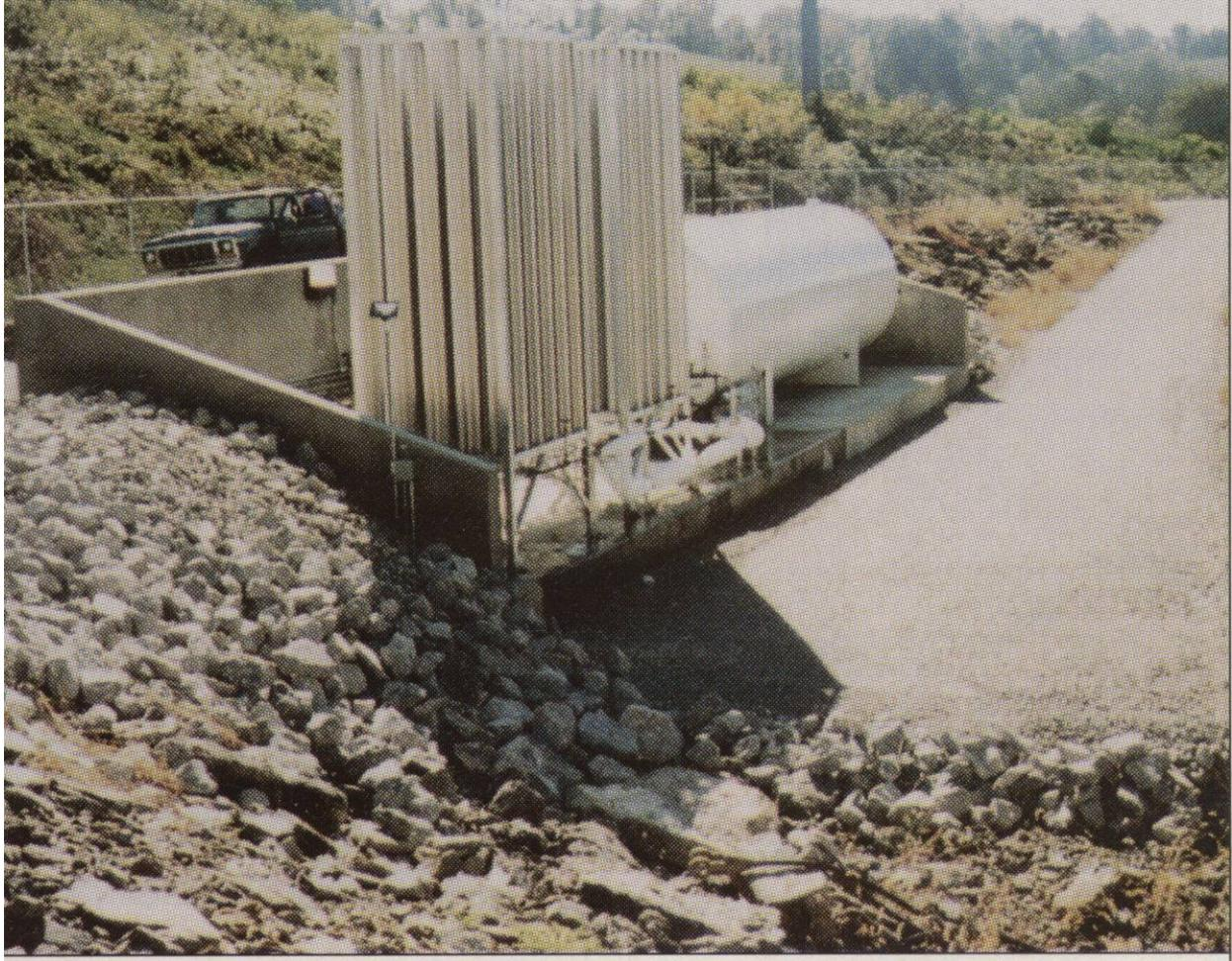
**Figure 4-6. Oxygen facility at TVA Tims Ford hydropower project**
