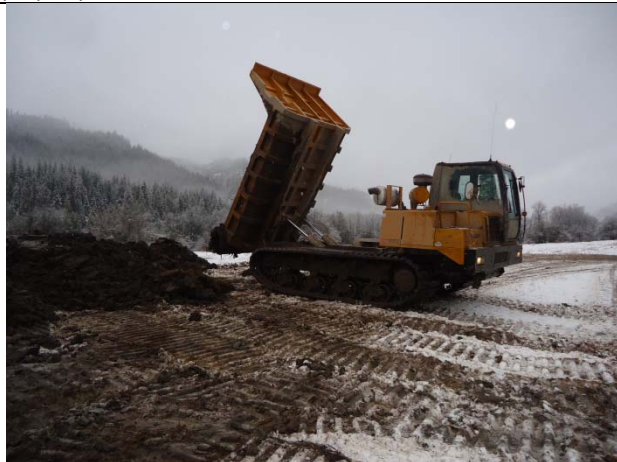
Photo 7. December 12, 2012. During construction. Dump truck moving earth from the excavations to the upland areas. Spoils were graded and seeded the following year, and planted with trees and shrubs.
