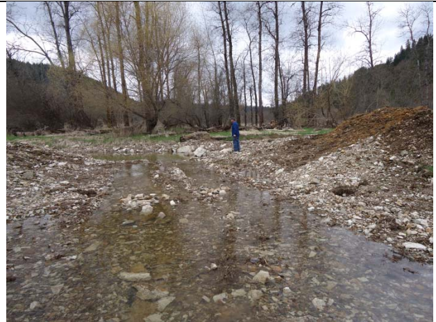
Photo 12. April 11, 2013. Outlet of the easterly Avista/IDFG property to the St. Joe River. Constructed rock spillway diverts water to the St. Joe river when it rises above a certain elevation at this location. On this date, water was at the planned maximum water surface elevation (Photo 11) and was overflowing to the river as designed.
