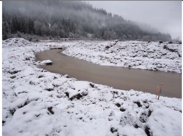
Photo 6. December 12, 2012. During construction. Swale created before removal of the large levee and ditch.
