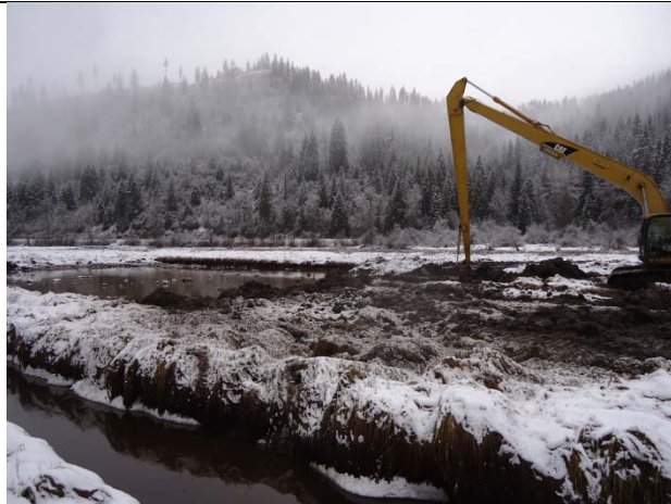
Photo 5. December 12, 2012. During construction. Long-reach excavator excavating one of the depressions on the Avista property.
