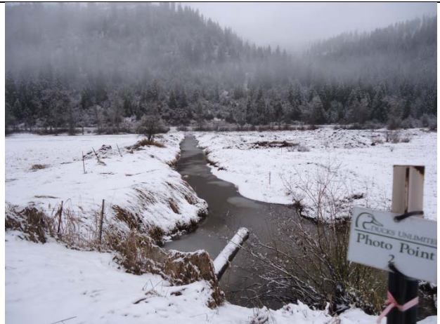
Photo 8. December 12, 2012. During construction. Levee and ditch features still remain. They were the last to be removed, so that a water control structure could be installed.
