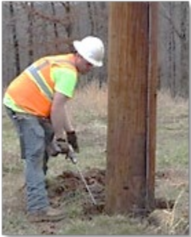
Wood Pole Inspection
