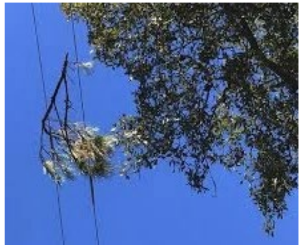
A branch spanning two conductor segments for a sufficient period of time may ignite the branch and also may produce high-energy, high-temperature arc
