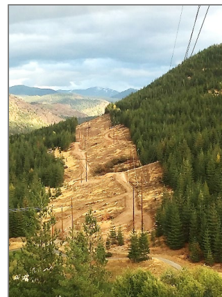
Avista Transmission corridor
