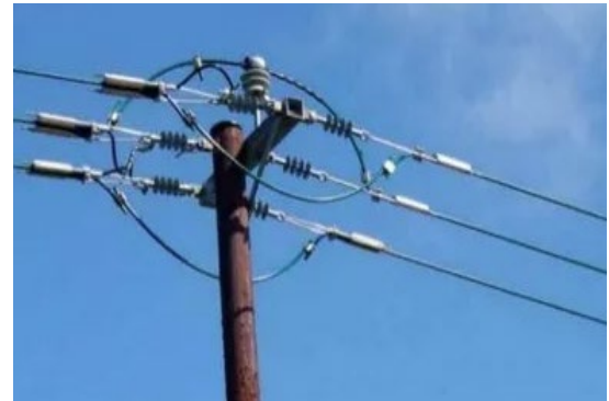
Covered Conductor is heavier and more robust than traditional bare wire.
