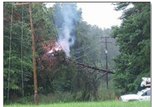
Example of a tree fall-in contacting power line
