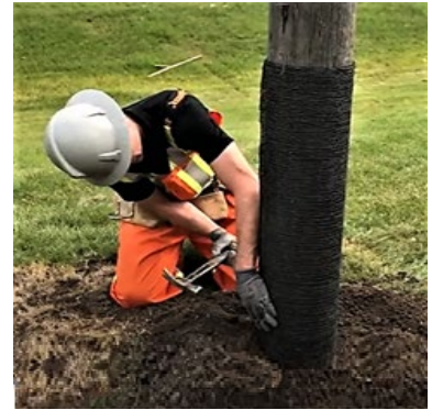
Installing fire resistant mesh wrap
