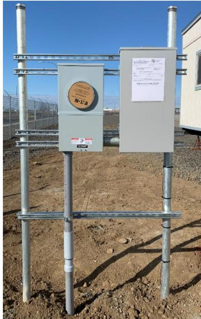
For residential only, a wood post embedded in concrete may be used for 200A meter pedestal in lieu of the rigid steel pipes and unistrut. Wood posts must be either a commercially new 6" x 6" treated post or a minimum 8-inch top diameter butt treated cedar or full treated white wood pole as depicted below.
