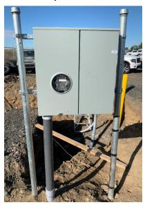
Figure 33 - 400 A Pipe Meter Pedestal Install Photo
