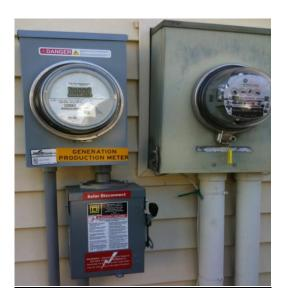
Figure 41 – Generation Production Meter and Disconnect Location
