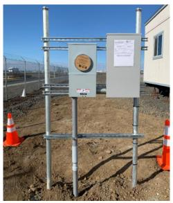
Figure 31 - 200 A Pipe Meter Pedestal Install Photo
